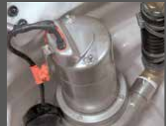
Pump with float switch
