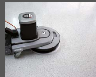
Polishing the PVC floor
