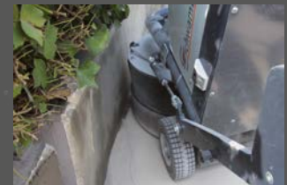
Grinding close to the edge with the remote control
